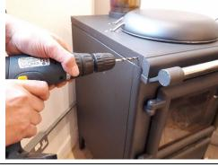
3. Using a 5mm drill bit, drill through the two marks on the side of the cookstove, to create the two fixing points.
