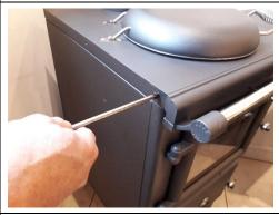
5. Loosely screw the supplied 2 x M6 bolts into the two fixing points.
