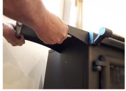
2. Use a pen or pencil to mark the position of the two fixing points on the side of the cookstove, through the two keyhole slots on the shelf.
