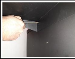
7. Tighten the two fixing bolts, so the shelves are held securely in position.
