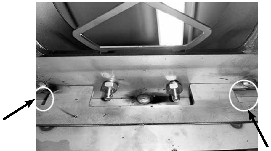
Figure 30. Front mounting slots for Flue Gas Agitator
