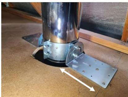
Each support wing is pre-drilled with 9 holes Each support wing spans 200mm
