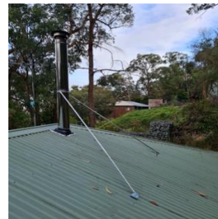
Supplied with 2 x support legs that adjust from 1,800mm up to 2,400mm in length
