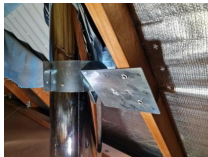
Adjustable support wings allow you to adjust the angle to brace to cross timbers
