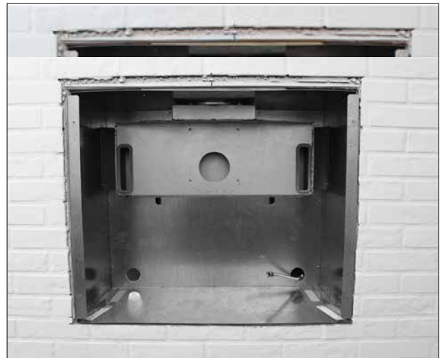
Zero clearance box and coaxial flue adapter
