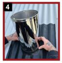
Put the ProFlash tape along the pipe ensuring there are no gaps between the ProFlash and the pipe
