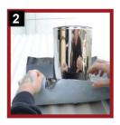
Put the ProFlash over the pipe and peel off the perforated backing from left to right
