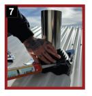
Apply the sealant and form the flashing to the roof profile
