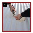
Cut the roofing sheet for the pipe size (size chart provided). Put the pipe in the hole
