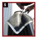
If required, cut the flashing to the pipe size
