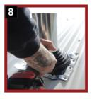
Start with screwing one vertical edge and then move across with the screws being between the valleys
